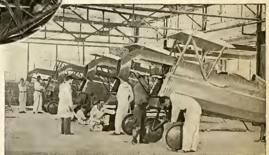
Students receiving instruction on engines, fuselage welding and the rigging of completed ships
